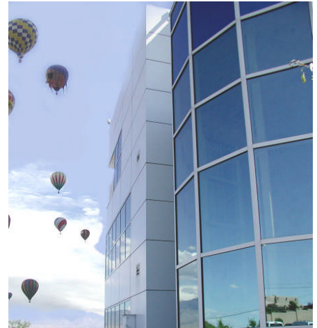
ECI's corporate office building received a Buildy Award for best integration project in North America.
