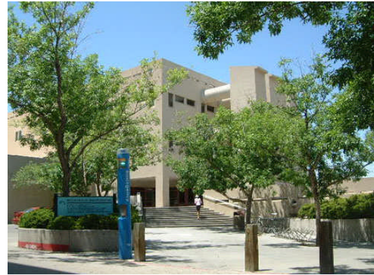
Mechanical Engineering Building
